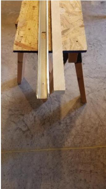
This shows the ripped 2 x 4 that fits into the metal stud.
