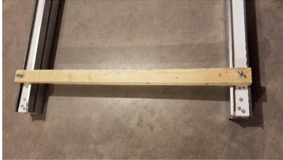
You should notice that I cut boards to fit into the rails. This gives more weight and keeps the rails lying flat (metal studs are very flimsy, but straighter than wood and have less friction than wood). I drilled the metal studs and wood, then used small bolts to fasten the rails together.
