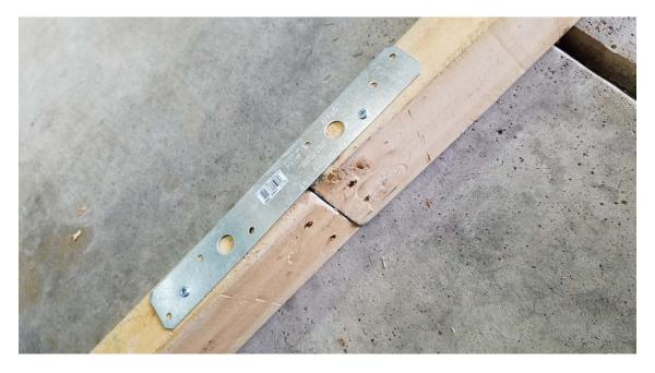
4. Use the steel angles and wood screws to secure the side rails to the end spacers.
